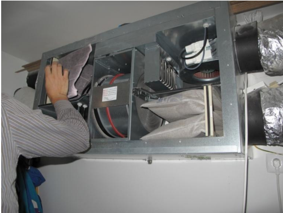
Plate 43. The heat exchanger for used air in the house of Rok Korenjak at Nova vas. Damjan Knap, ( http://nep.vitra.si/ukrep.php?h=knap&id=41 ) at Cerknica built a new house, passive heating, under floor heating with a rainwater storage system. (Plate 44).
