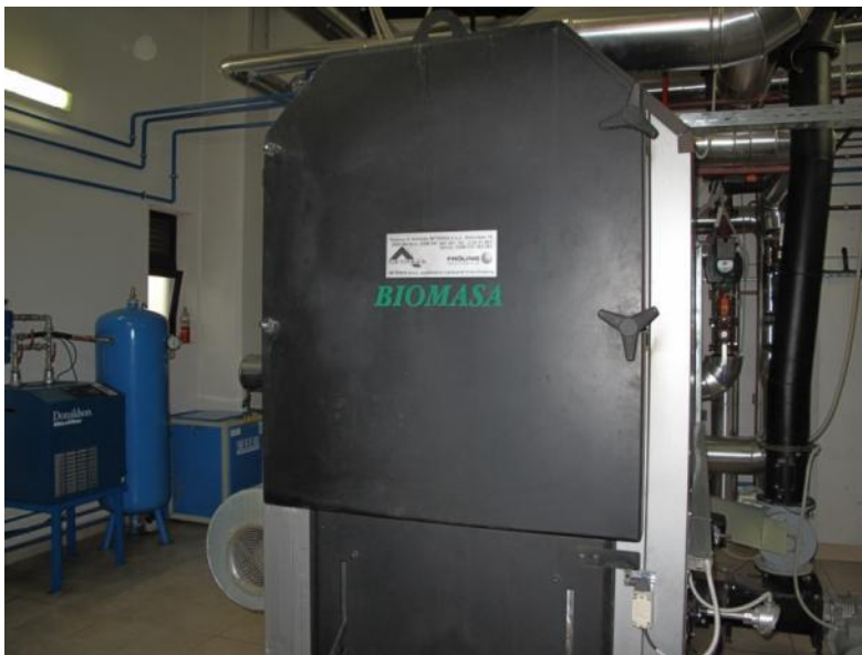
Plate 12, The boiler 220 kW used to heat the Okna Šemrl factory using self generated wood waste.
