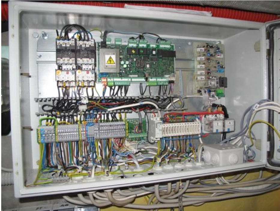
Plate 37. Microprocessor controls and circuitry used to control the smart house of Uros Mihelic.
