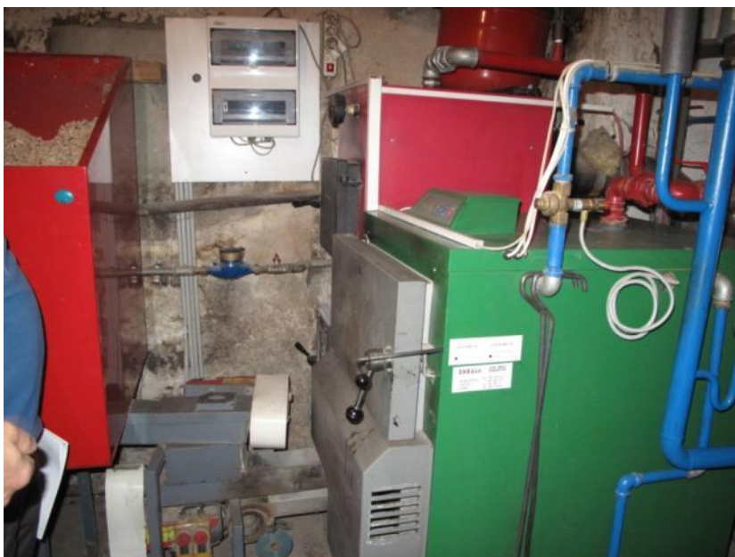
Plate 34. Home modified wood chip boiler with auto feed.
