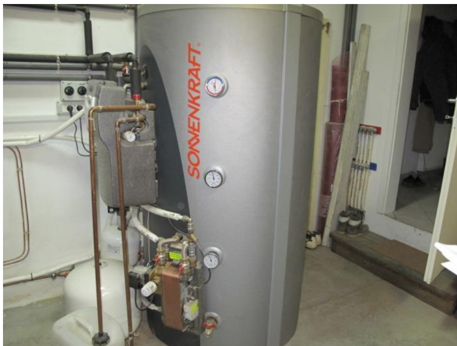
Plate 56. Heat exchanger for hot water system in the house of Igor Blažina.
