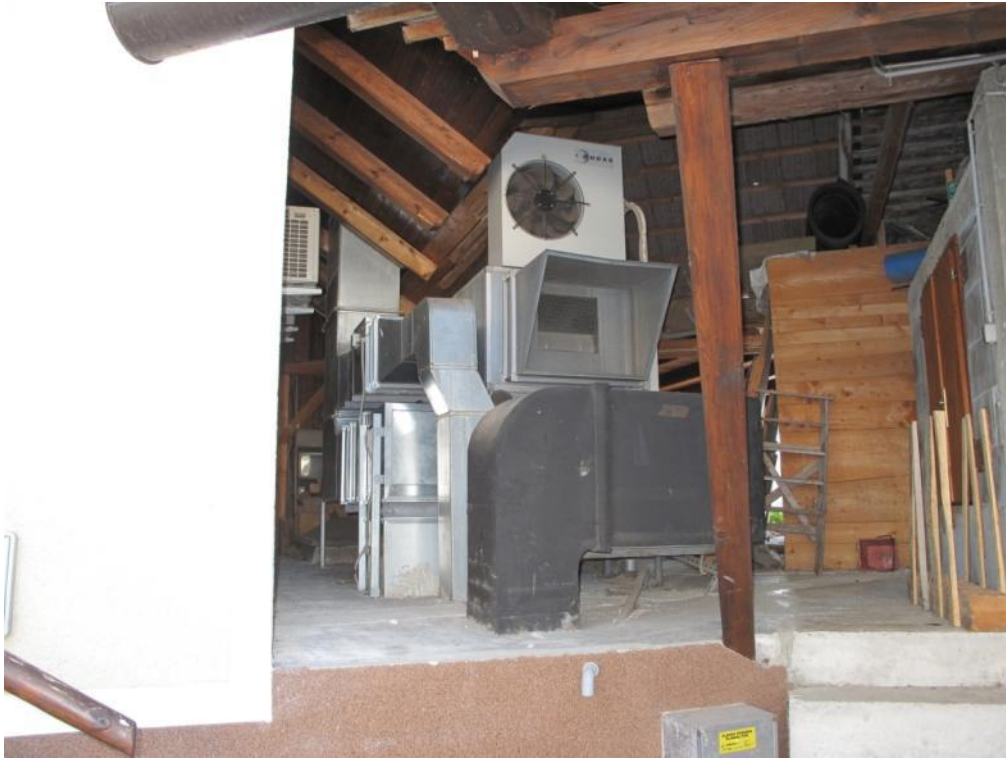
Plate 23. Air heat recovery from the Gostilna Turk at Hotedršica.
