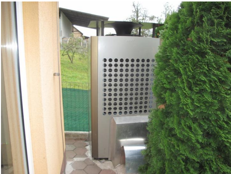
Plate 38. External heat pump drawing air from a pre-warming underground pipe prior to extracting heat.
