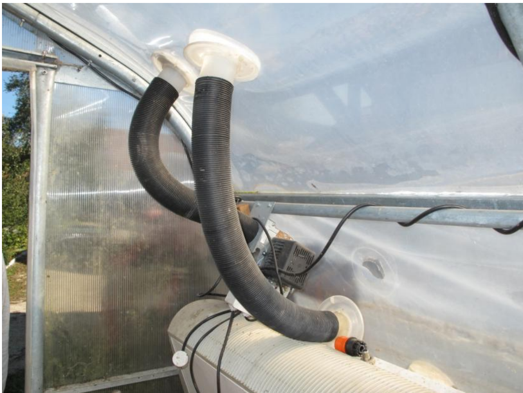
Plate 24. Air fan system to separate layers of polyethylene to give a thermal barrier in polythene tunnel house to produce vegetable for the hotel Gostilna Turk at Hotedršica.
