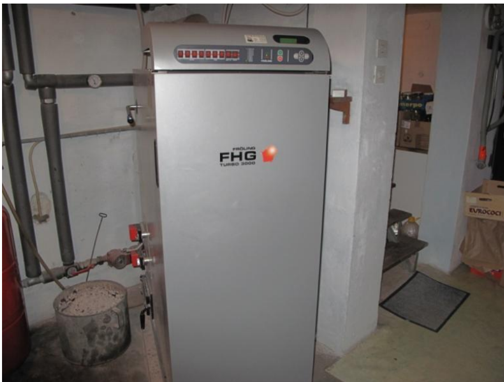
Plate 26. Logwood boiler for house / cafe/ distilling plant.
