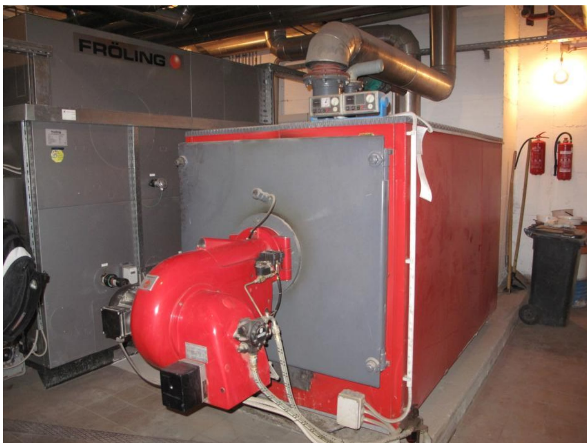
Plate 17. The chip burning plant at SGLŠ.
