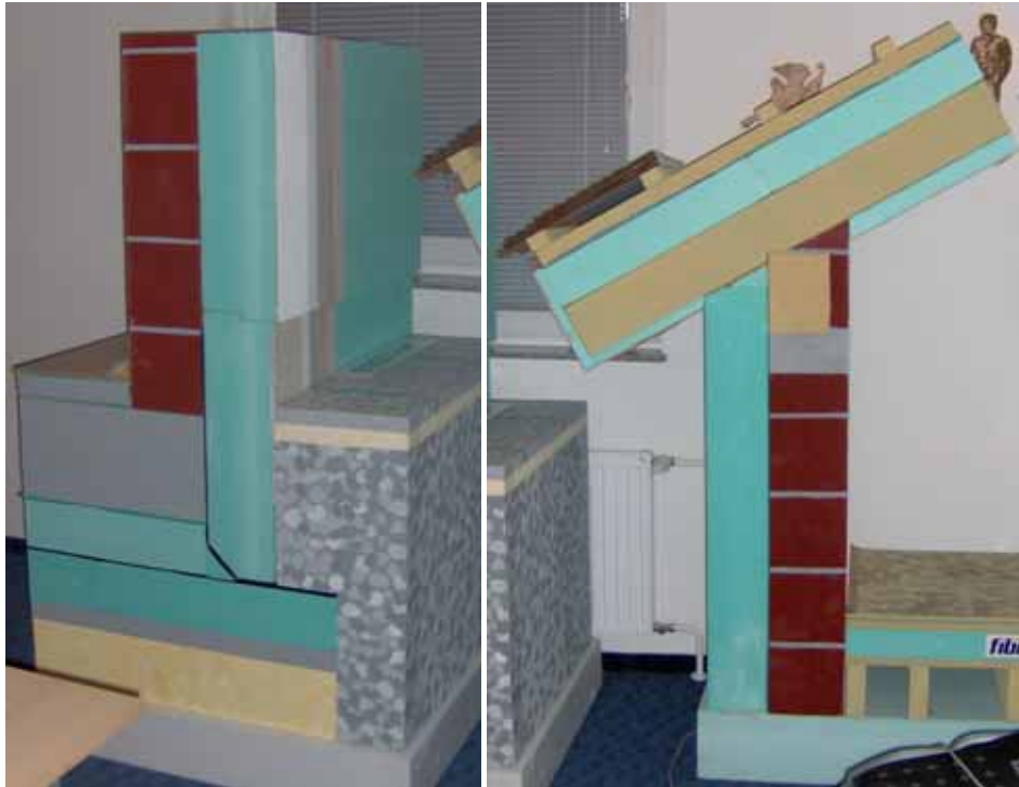
Wall and roof insulation model showing use of expanded polystyrene
