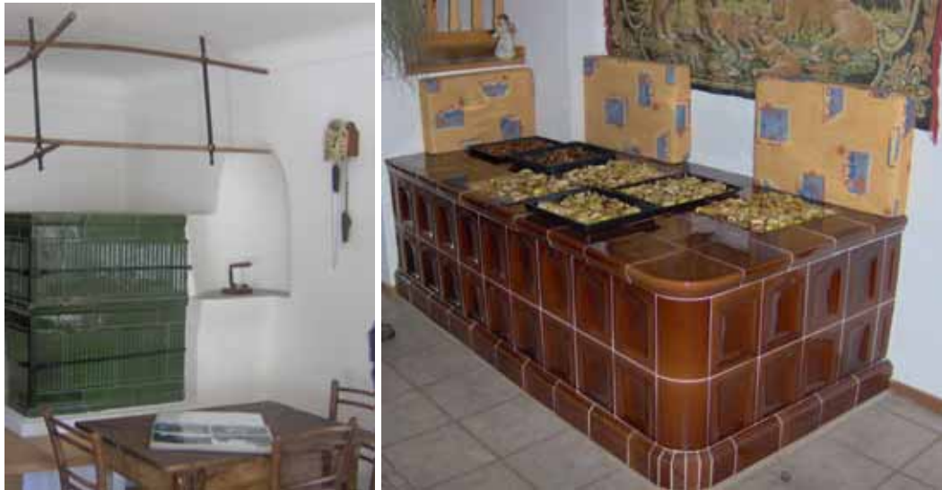
A traditional Slovenian heating system and a unit retained in a refurbished house
