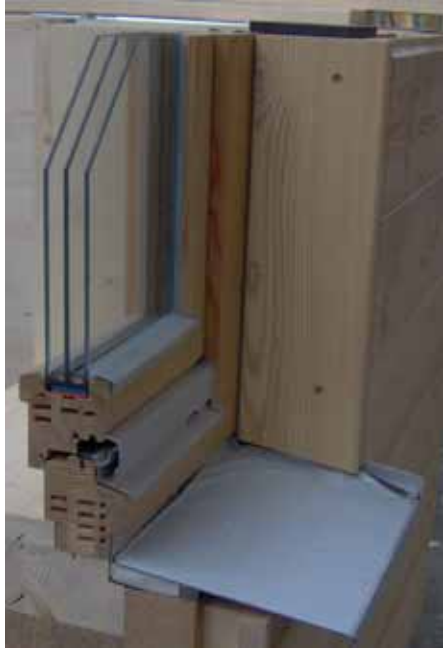
Section through triple glazed window
