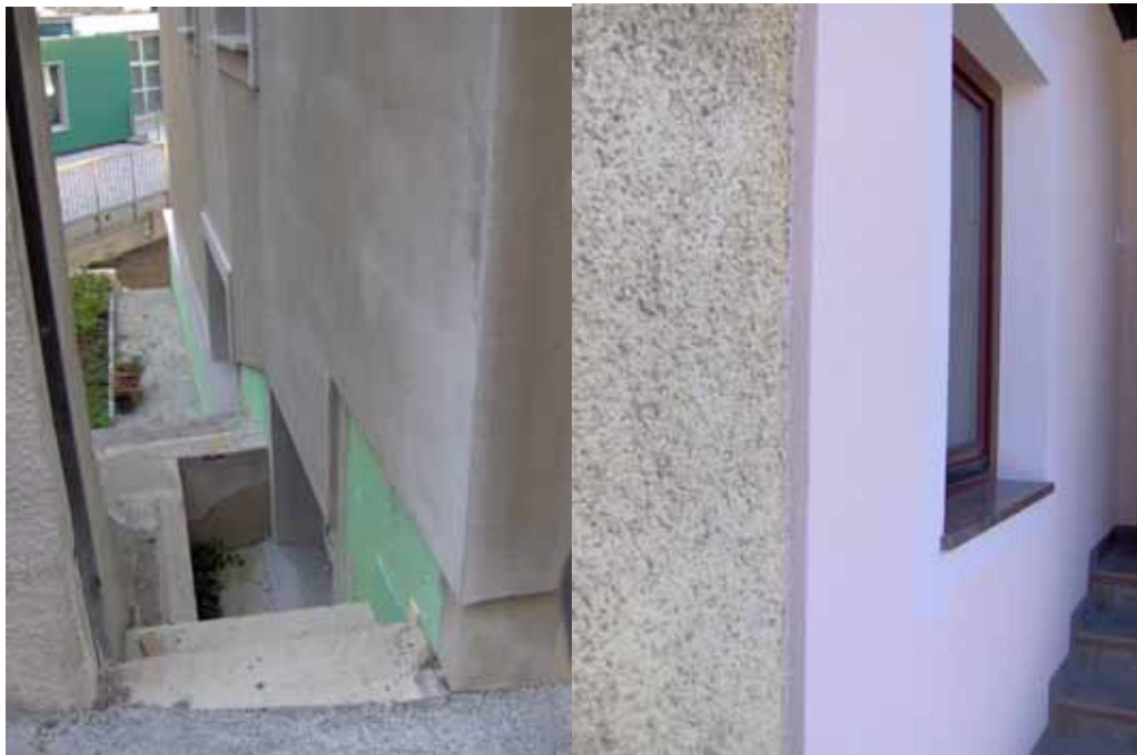
External Insulation and Re-rendering
